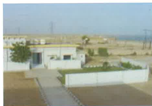
Fig. 5. SWRO Plant at KANUPP, Pakistan.
