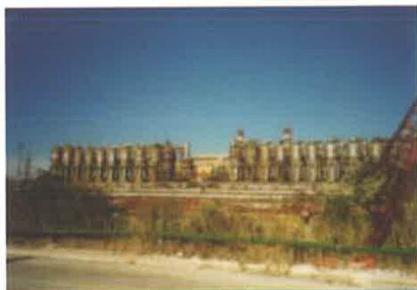
Fig. 2. Evaporators at Aktau, Kazakhstan.
