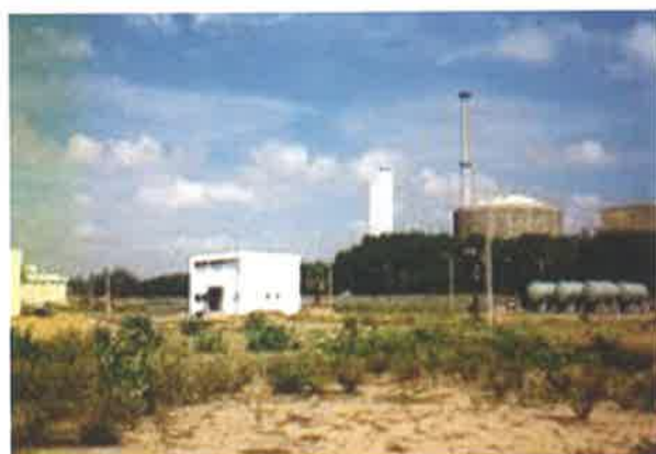
Fig. 4. Hybrid (MSF+RO) plant, Kalpakkam, India.
